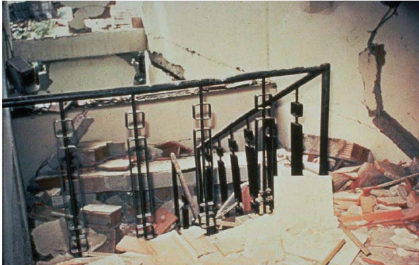
Figure 1.11: Undesirable earthquake performance of elements assumed to be non-structural elements during 1972 Nicaragua Earthquake: Damage to unreinforced masonry infill and floor tiles around stairwell (Photo: The EERI Annotated Slide Collection, 1997)
