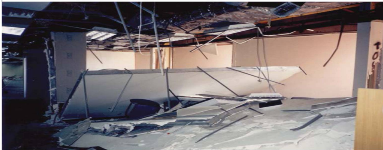
Figure 6. (above) Partition tipped over, 1994 Northridge Earthquake. (bottom) Fallen stud/gypsum board partition, source: Wiss, Janney, Elstner Associates, FEMA 74 From [14]
