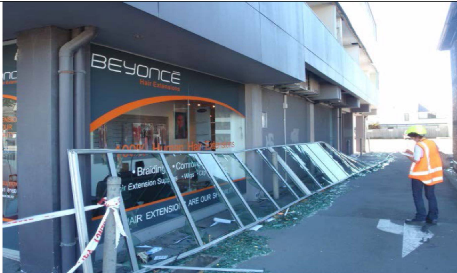
Figure 1. Widespread damage to a glass ceiling system From [18], H. Ferner, M. Wemyss, A. Baird & A. Beer, Seismic performance of non-structural elements within buildings
